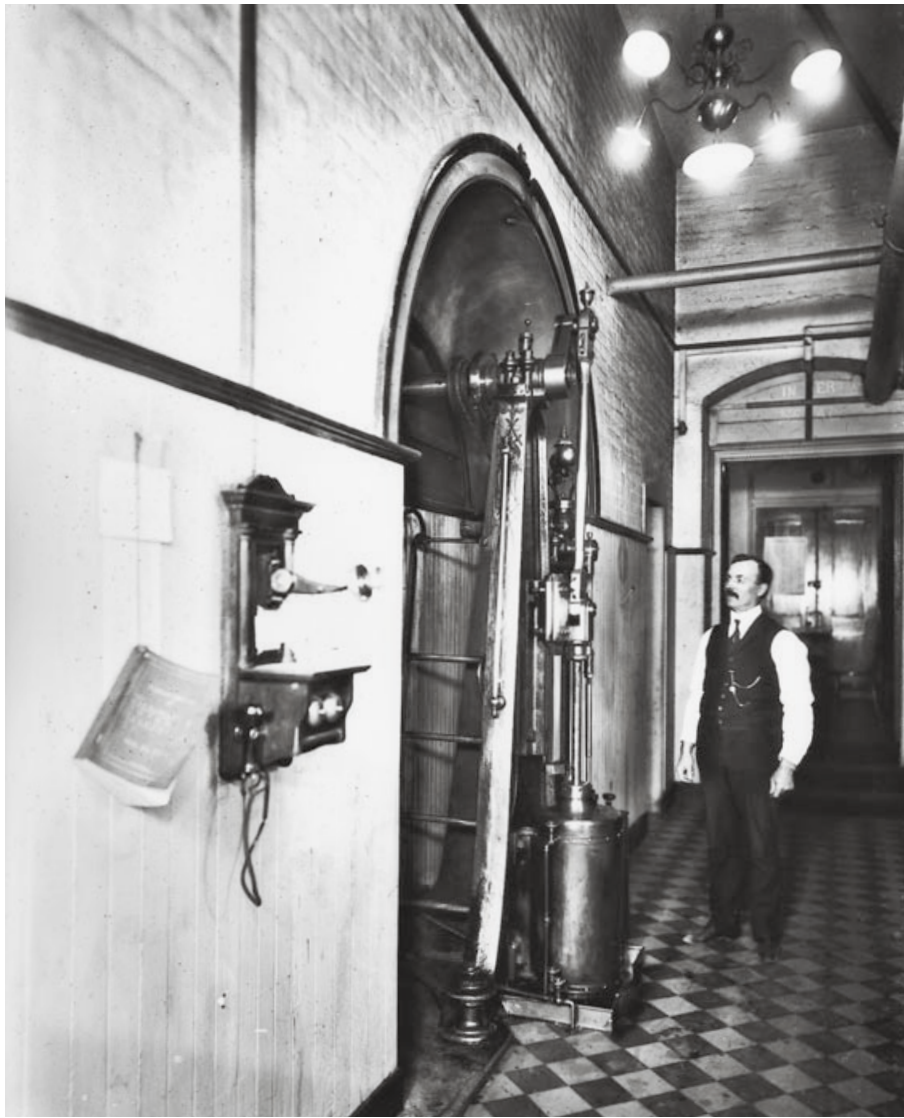
Steam Engine and Fan ca. 1911
