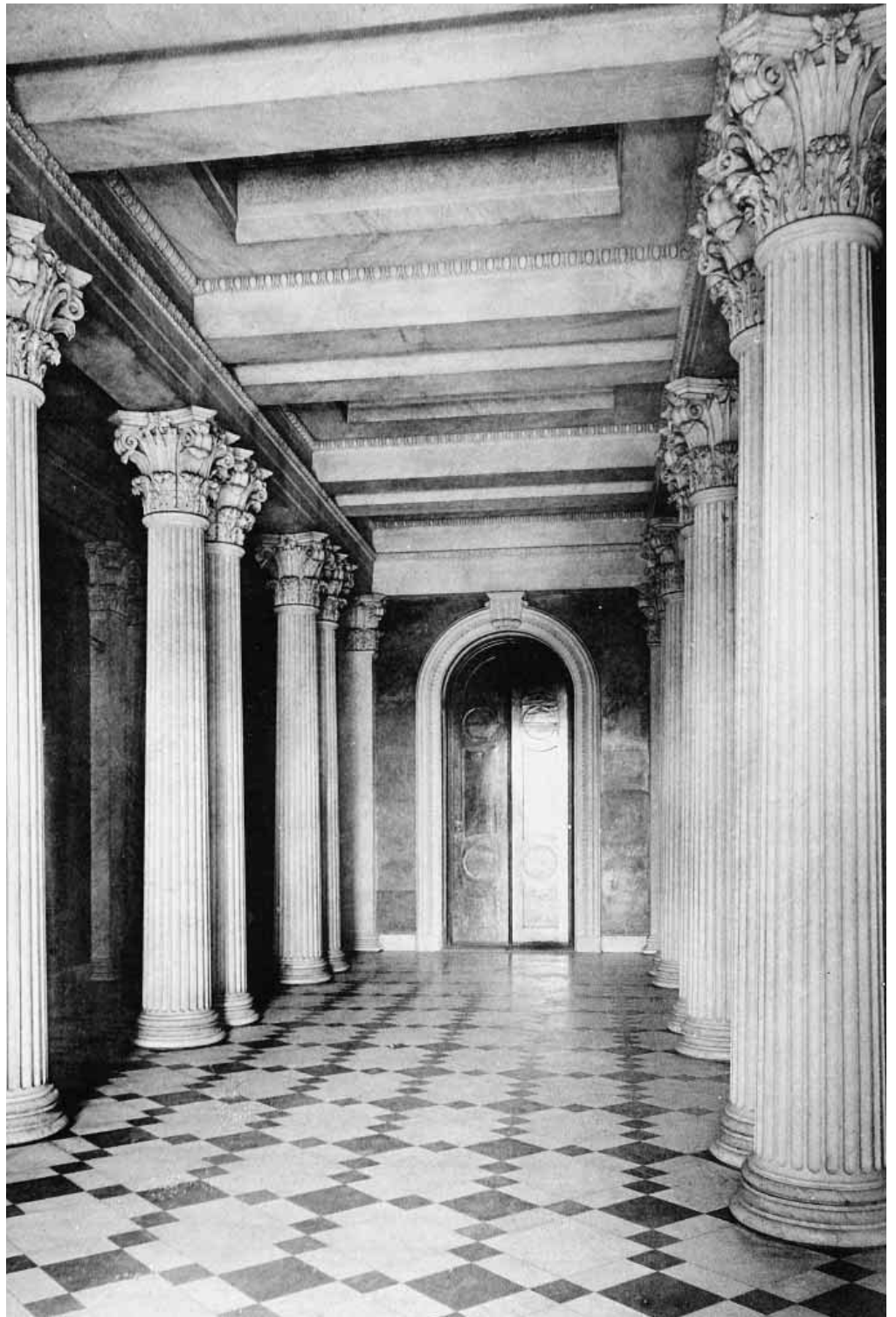
Fig. 4–9. Senate Corridor, Principal Story, c. 1902. For the main passage into the Senate Chamber, Walter designed a heroic double colonnade of paired Corinthian columns supporting a richly carved marble ceiling with stained-glass panels. Walter incorporated tobacco, corn, and magnolia leaves in the capitals.
