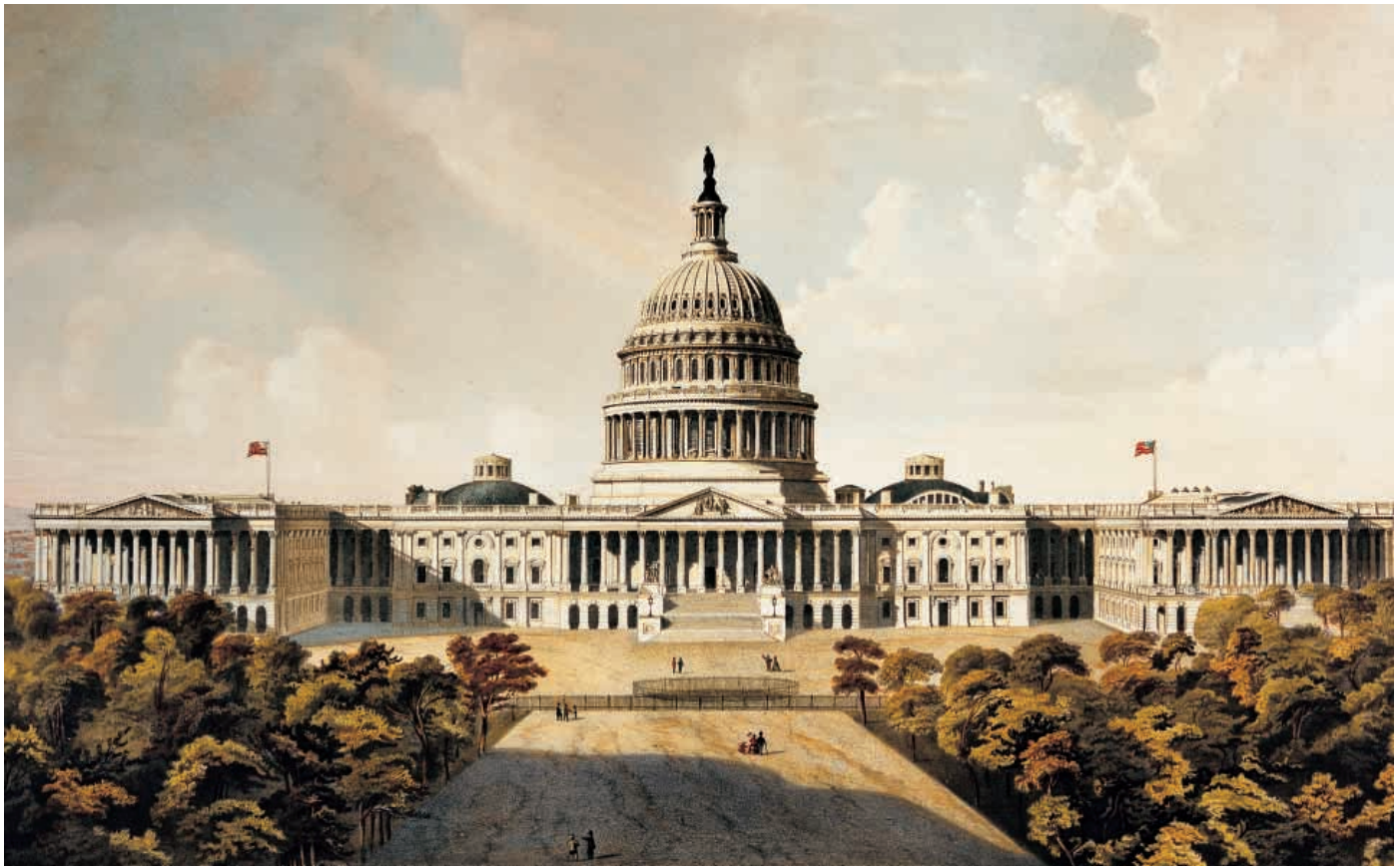
Fig. 4-3. Charles Hart, U.S. Capitol Washington, D.C., c. 1866. Although differing in detail and materials, the two wings that were added to the Capitol were designed to harmonize with the existing structure. The great cast-iron dome, completed in 1866, unified the composition. U.S. House of Representatives, Conable Collection.
