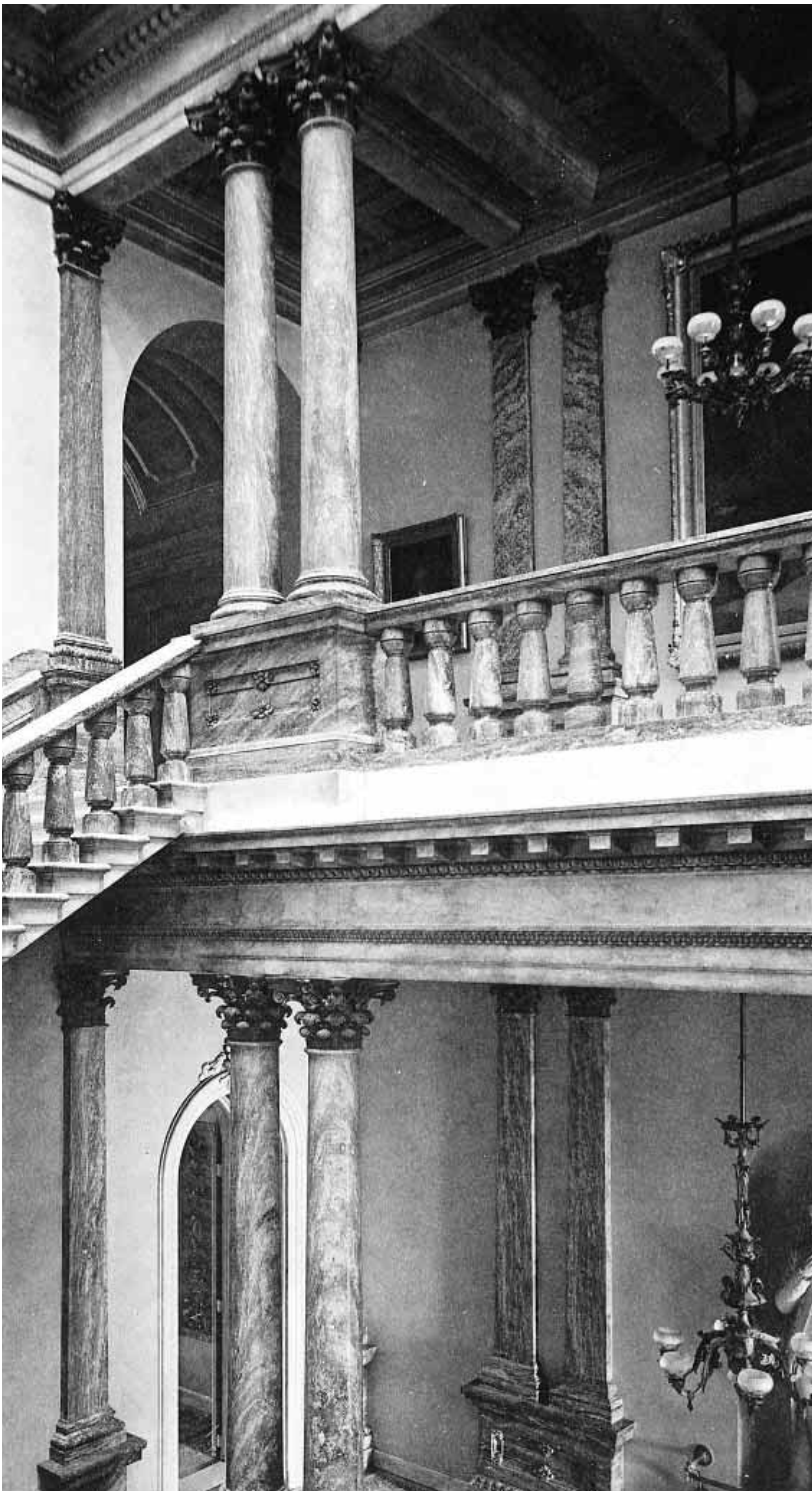
Fig. 4-10. East grand stair, House wing, c. 1902. Each wing was provided with two monumental public stairs designed with Corinthian columns and pilasters with bronze capitals, massive handrails and balusters, steps carved from individual blocks of marble, and niches for sculpture.
