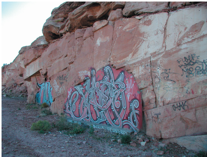
Figure 3. Concrete-barricaded portals in Coconino Sandstone at the South Arden Quarry site.
