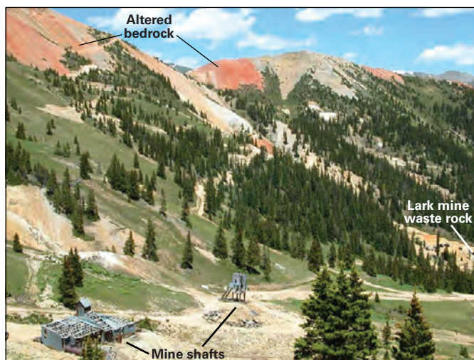
Figure 3. View of Prospect Gulch, looking north, with abandoned mines (acid-mine drainage) and areas with altered bedrock (acid-rock drainage).
