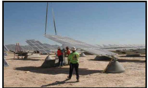
Tripod trackers are installed
