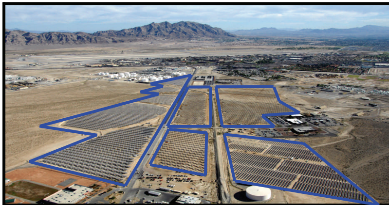
Aerial View of the Solar Array after Construction Completion
