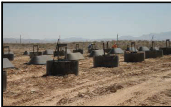
Non-invasive concrete foundations are cast
