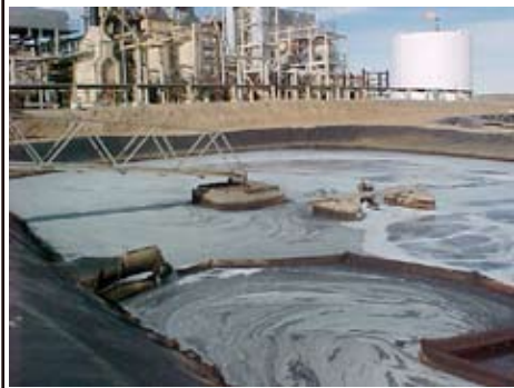
Discharging benzene to an aeration basin which is part of the wastewater treatment system. Non-NPDES volatiles were emitted from the SI. Benzene was found in the sediments in the basin. This resulted in a $75,000 penalty with injunctive relief involving installation of filtration and air stripper units.
