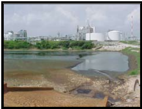
Emergency retention basin receiving overflow from the wastewater treatment plant. Vacuum trucks dump into the SI. Wood-lined ditches for wastewater conveyance. Methylene chloride had been spilled and routed to the base of the SI. Groundwater data was found to show methylene chloride at very high levels.
