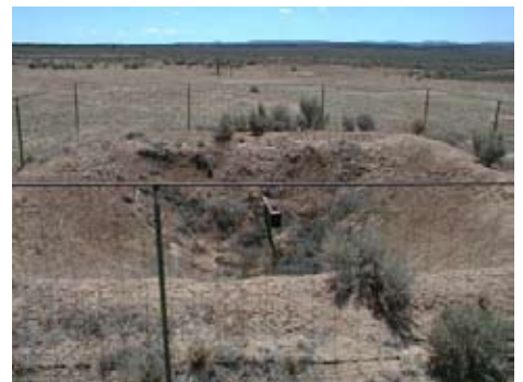
A ramp leads into the SI, which is not covered. It receives a mixture of wastes and D008 sludge.
