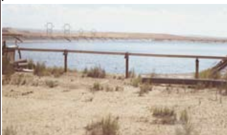
Coal fired power plant with 14 evaporation impoundments. 8 of these impoundments exceeded selenium hazardous waste levels. They failed to make waste determinations and did not have a permit for waste disposal.
