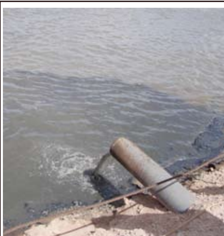
SI receiving discharges of benzene (5-20 mg/L). The facility was also found to have a leaking API separator that is also an SI. The facility has no NPDES permit.
