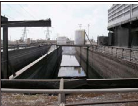
A ramp leads into the SI, which is not covered. It receives a mixture of wastes and D008 sludge.
