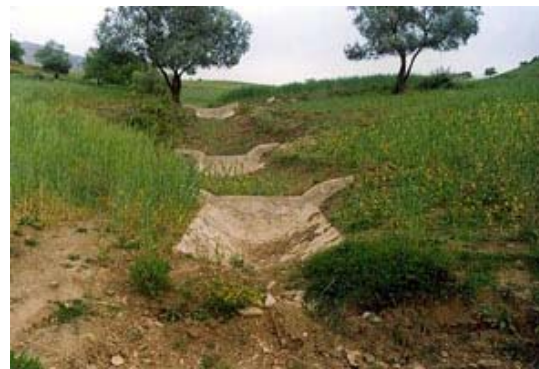
Figure 10.4 Best management practices are an integral part of USAID's sustainable agriculture program in Morocco. The project constructed check dams along this ravine to prevent erosion, thereby enhancing soil and water conservation.
