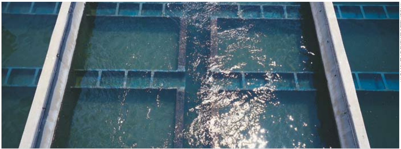
View of the clearator, Karang Pilang Water Treatment Plant II in Surabaya, Indonesia.
