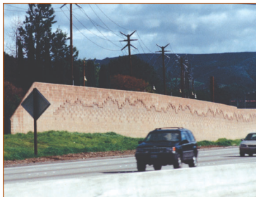
Noise barriers reduce the sound that enters a community from a busy highway. (Photo courtesy of Environmental Measurement and Modeling Division)
