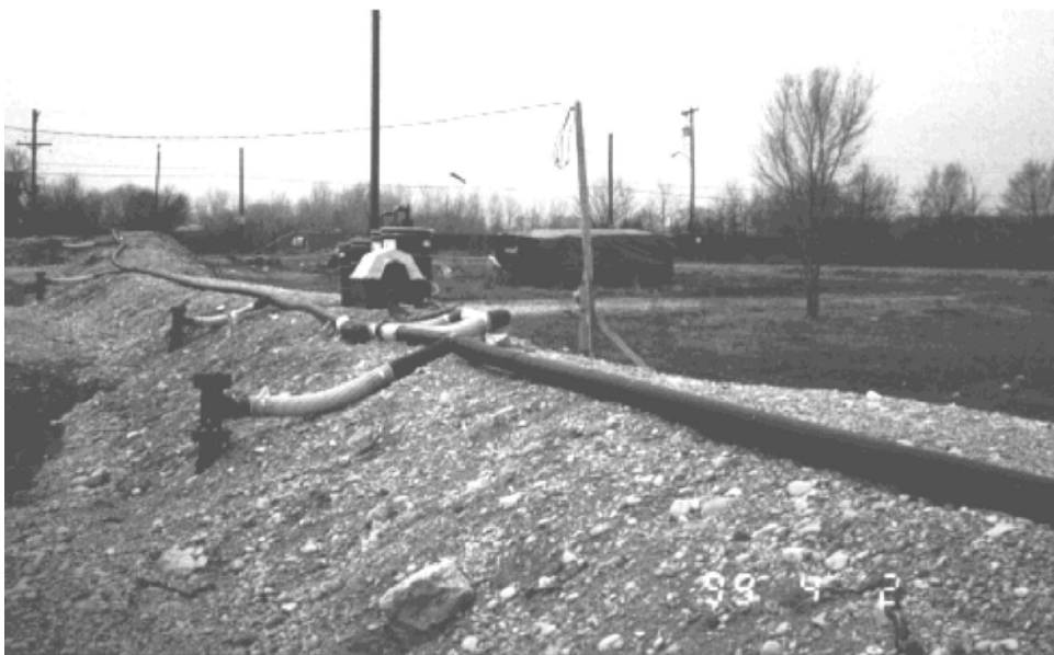
Figure 3-6. Alternative Migration Barrier System.
