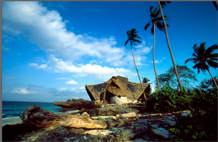
The visitor center takes advantage of trade winds to cool the facility. © Craig Zendel
