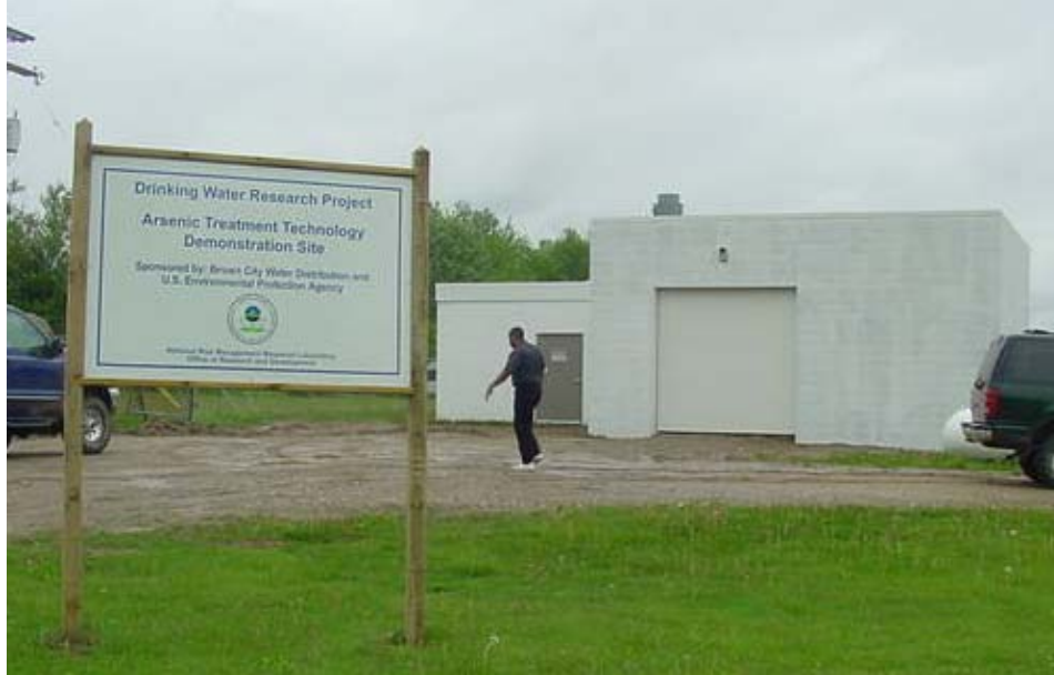
Figure 4-7. New Building Adjacent to Preexisting Pump House (on left)
