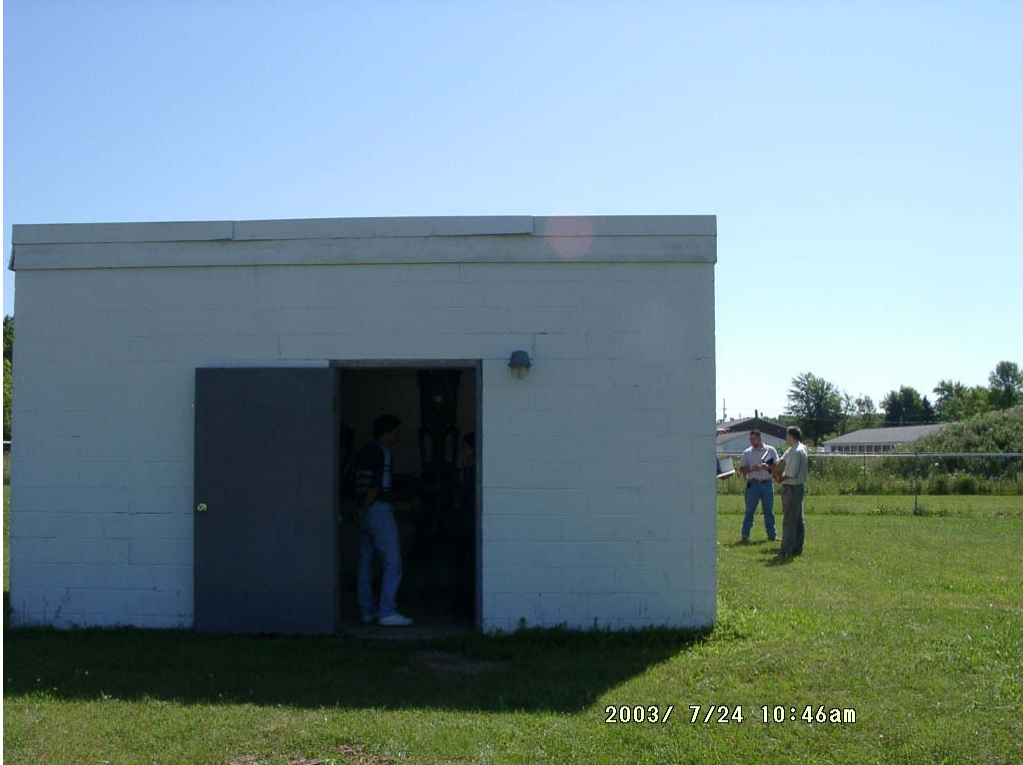
Figure 4-2. Former Well No. 4 Pump House at Brown City
