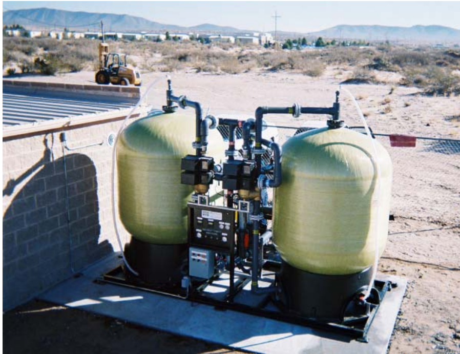
Figure 4-10. APU-300 System before Building Enclosure was Built
