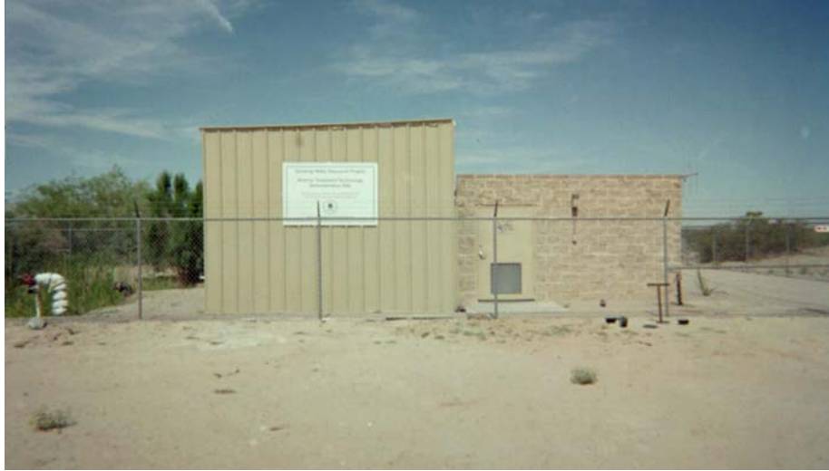
Figure 4-8. Pump House (right) and System Enclosure
