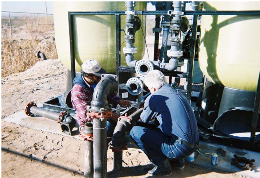
Figure 4-9. APU-300 System Being Connected to Distribution System
