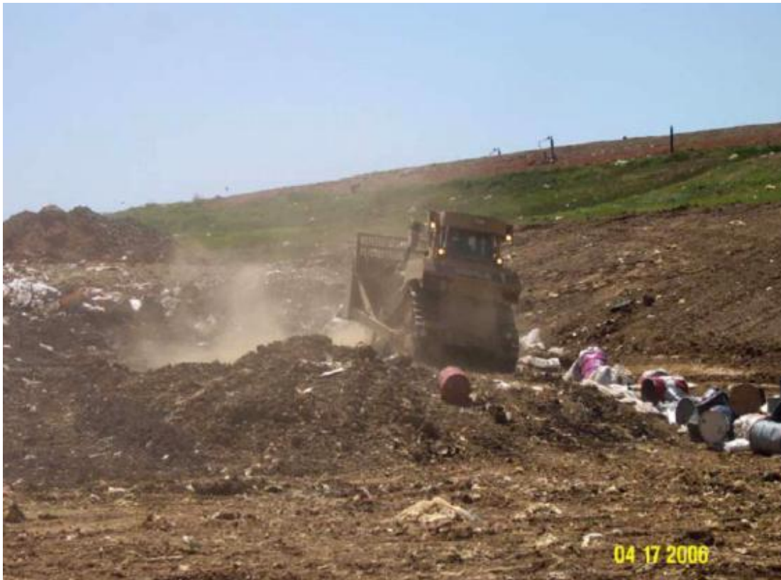
Figure 4-8. Covering abatement debris at the landfill.
