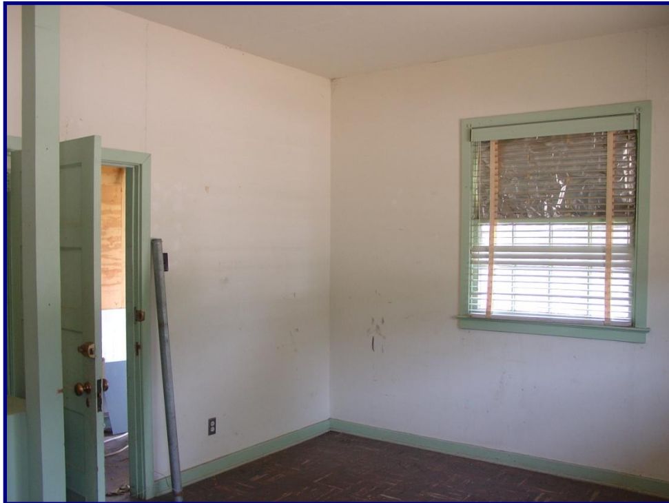
Figure 3-3. Interior view of Building #3602 (NESHAP). Interior finishes are gypsum wallboard (ceiling and walls) and nine-by-nine-inch resilient floor tile.
