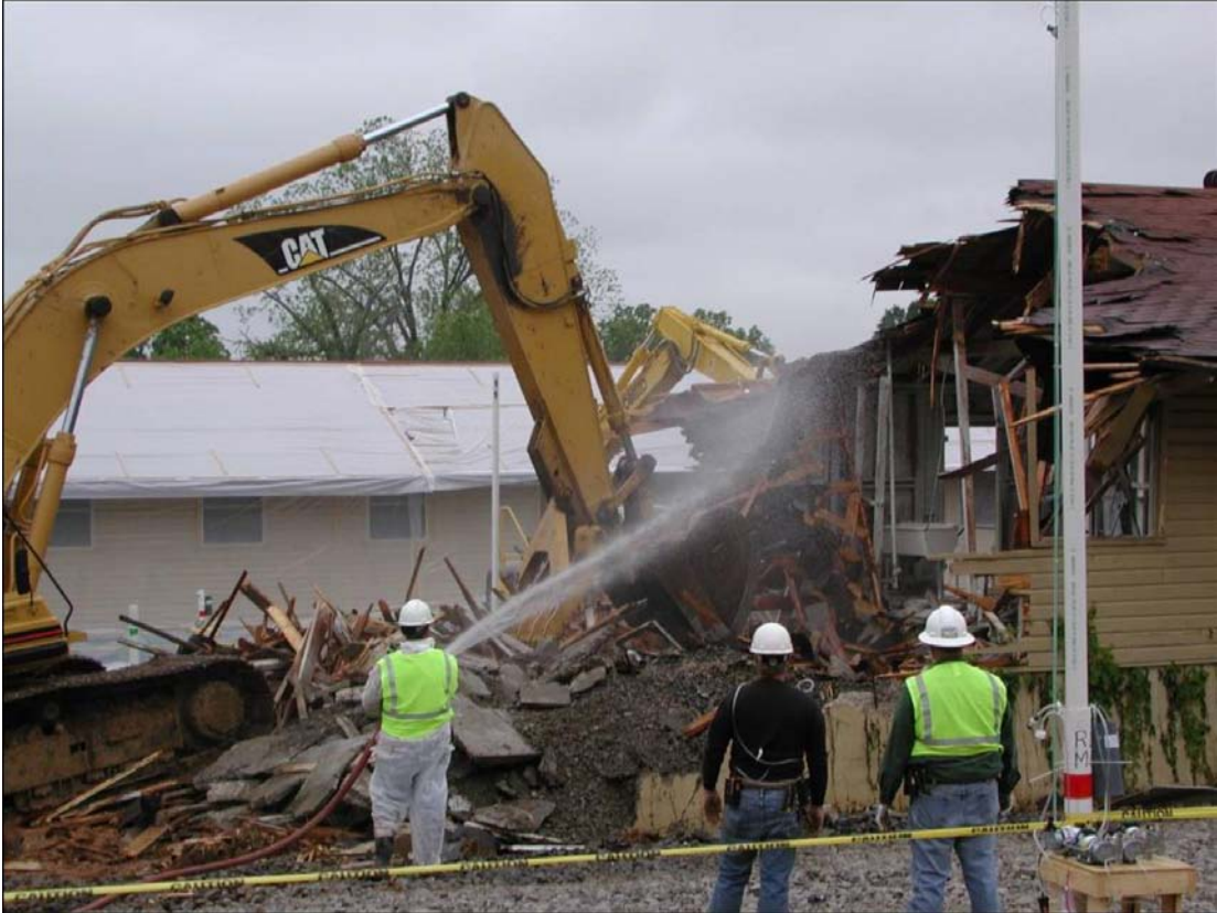
Figure 4-17. Starting demolition of the NESHAP building.
