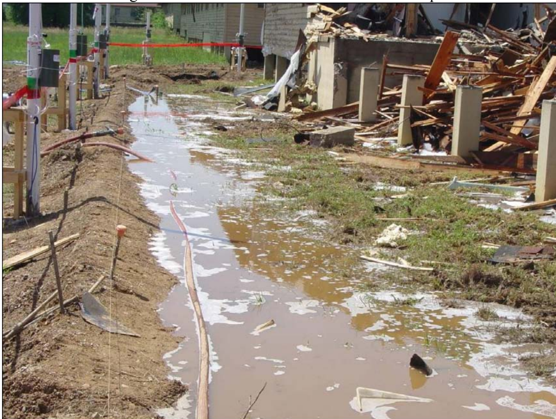
Figure 4-10. Water accumulation near the berm during the ACM demolition.
