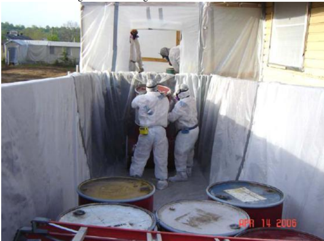
Figure 4-5. Loading asbestos-containing material into roll-off container.
