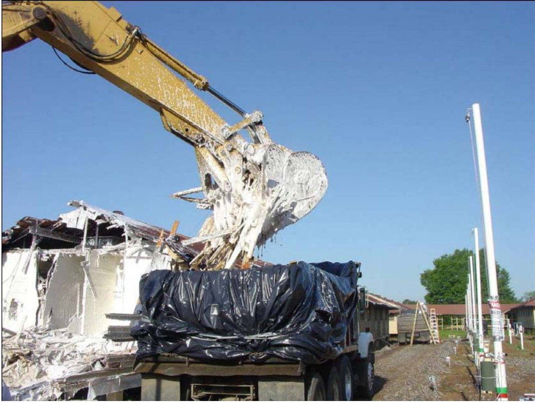
Figure 4-33. Loading the AACM demolition debris.
