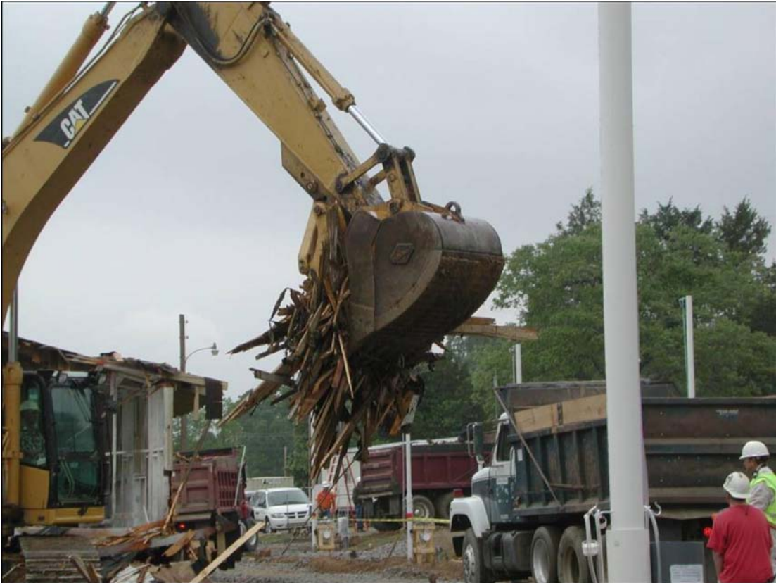
Figure 4-18. Loading NESHAP debris into trucks.
