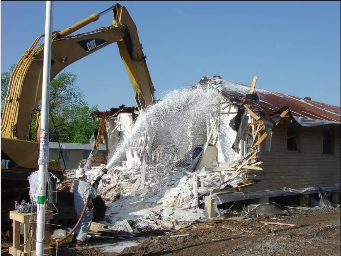
Figure 4-32. Progressing with the AACM demolition.
