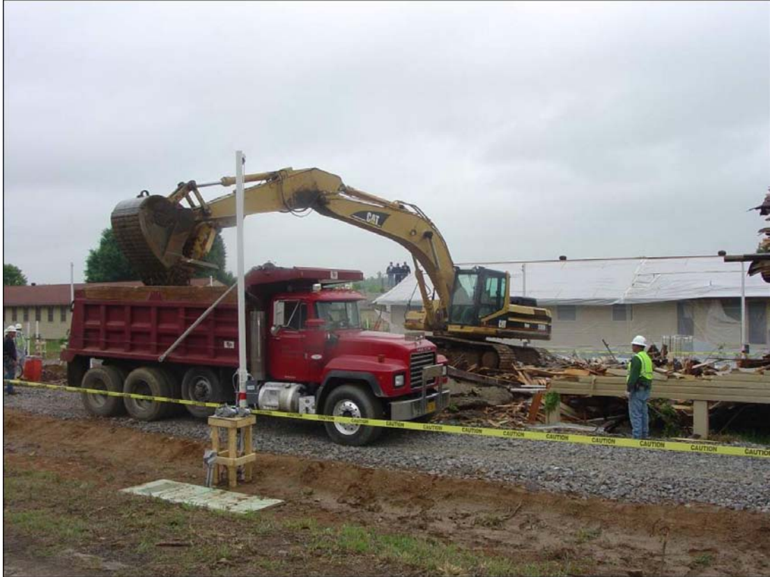
Figure 4-19. Finishing NESHAP demolition.
