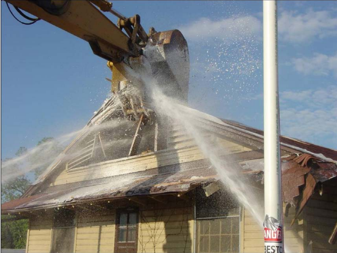
Figure 4-31. Starting the AACM demolition.
