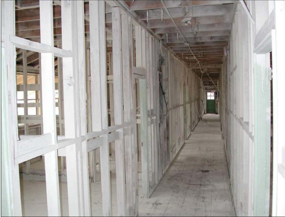
Figure 4-6. Abated area after application of encapsulant.
