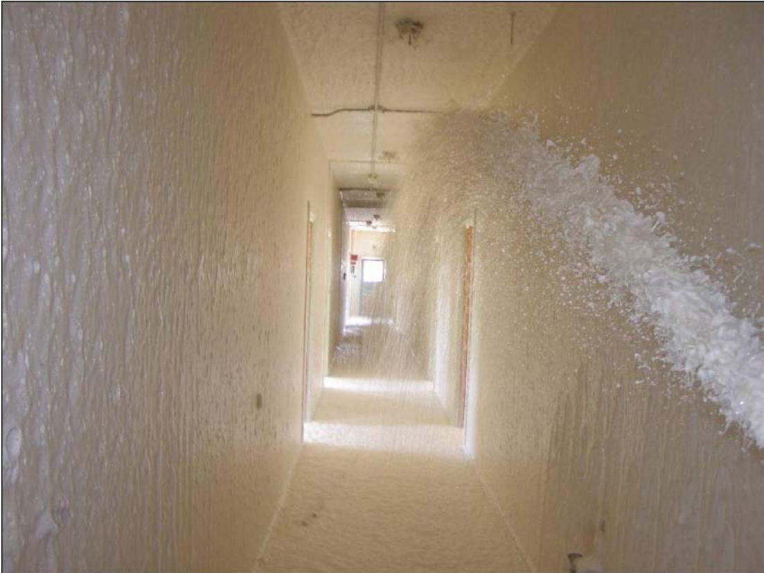
Figure 4-24. Pre-wetting the hallway with Amended Water.
