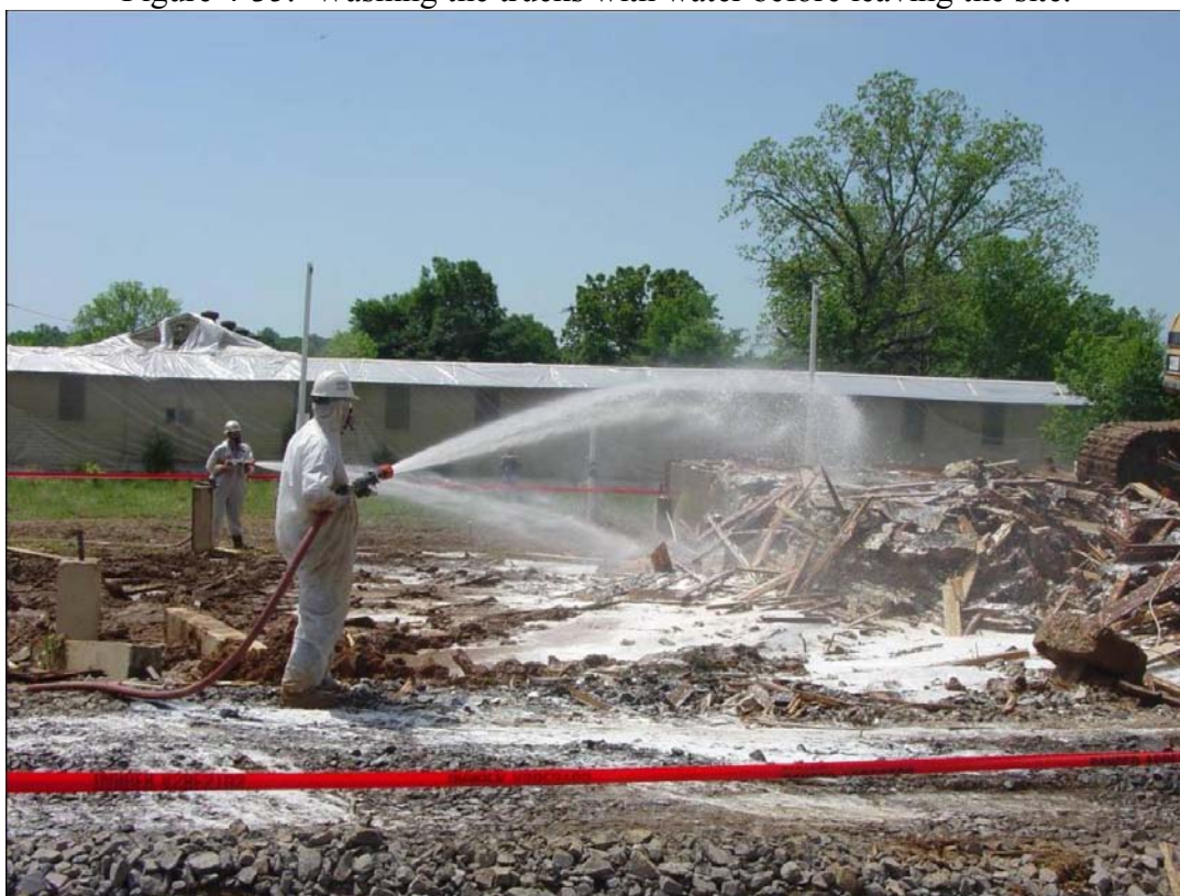
Figure 4-36. Nearing the completion of the AACM demolition.
