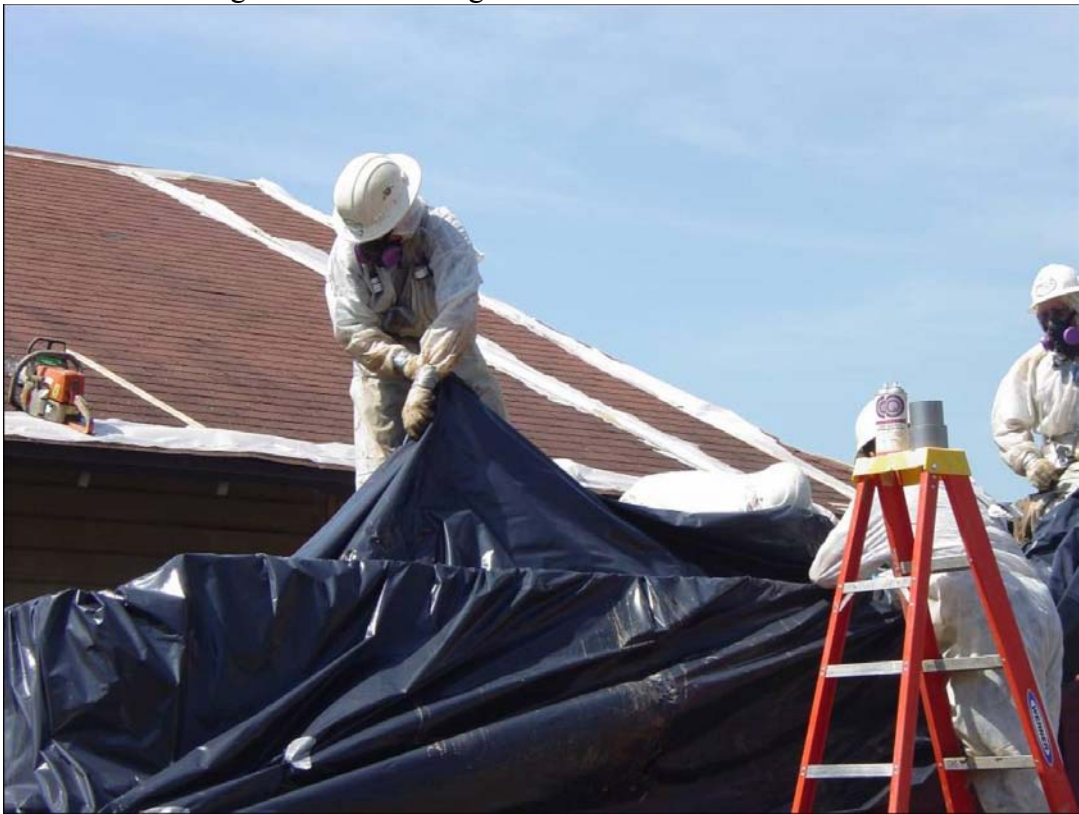
Figure 4-34. Sealing the “burrito wrap” before leaving the AACM site.
