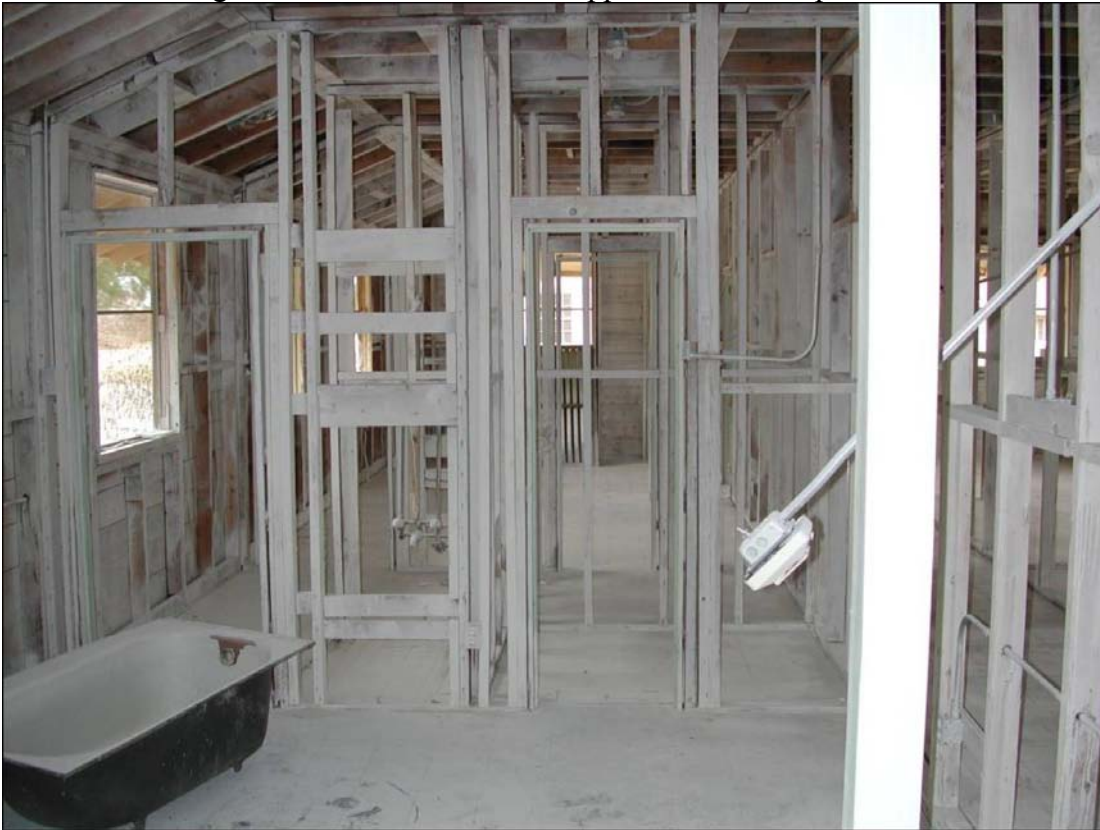
Figure 4-7. Abated area after final clearance.
