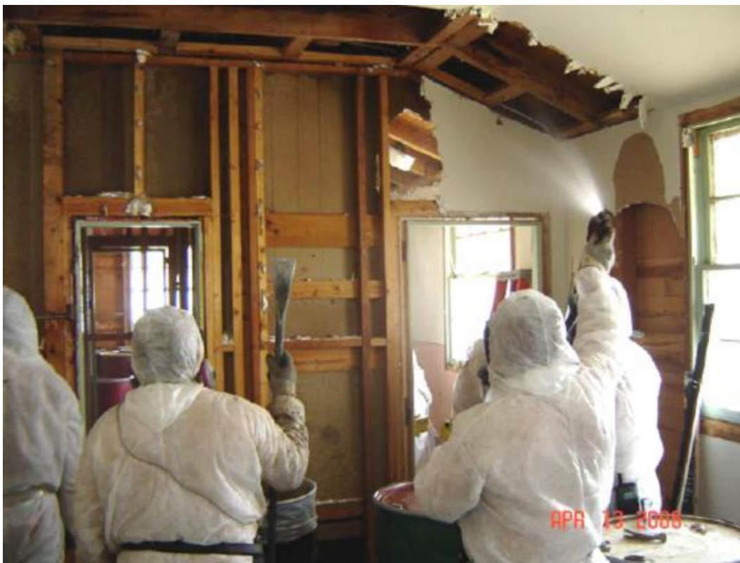
Figure 4-3. Wetting and removal of drywall during abatement of NESHAP building.
