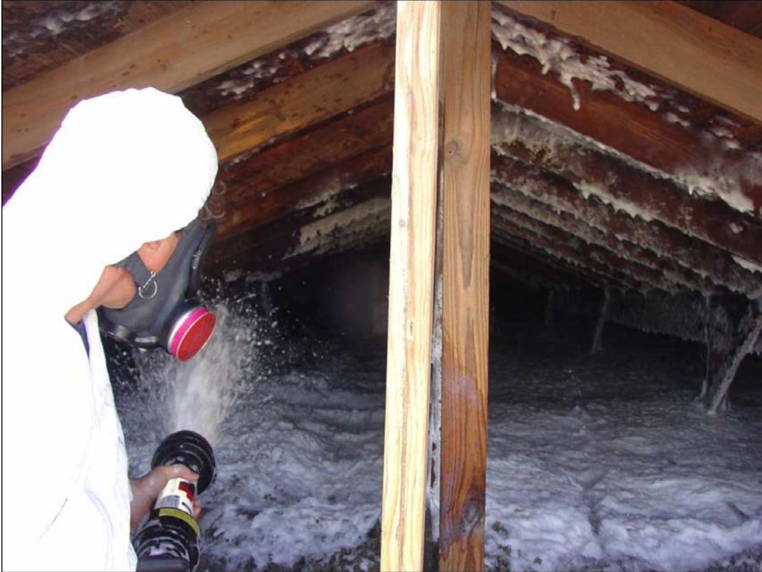
Figure 4-25. Pre-wetting the attic with Amended Water.
