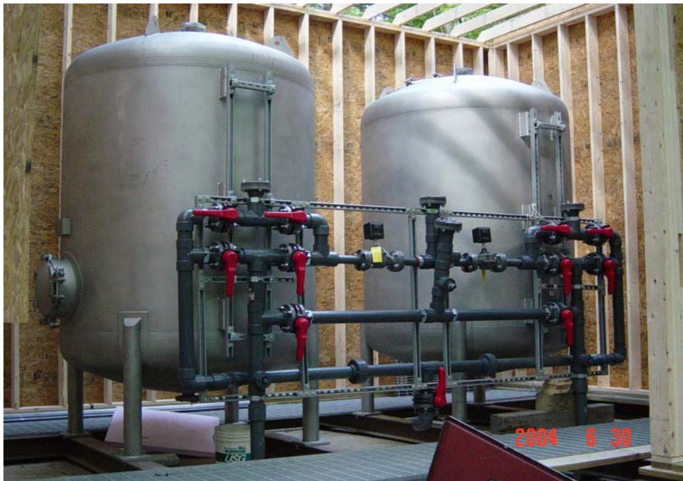
Figure 4-6. ADI G2 Media Arsenic Adsorption System
