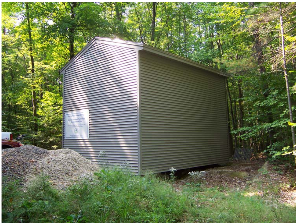
Figure 4-7. New Treatment Building Addition
