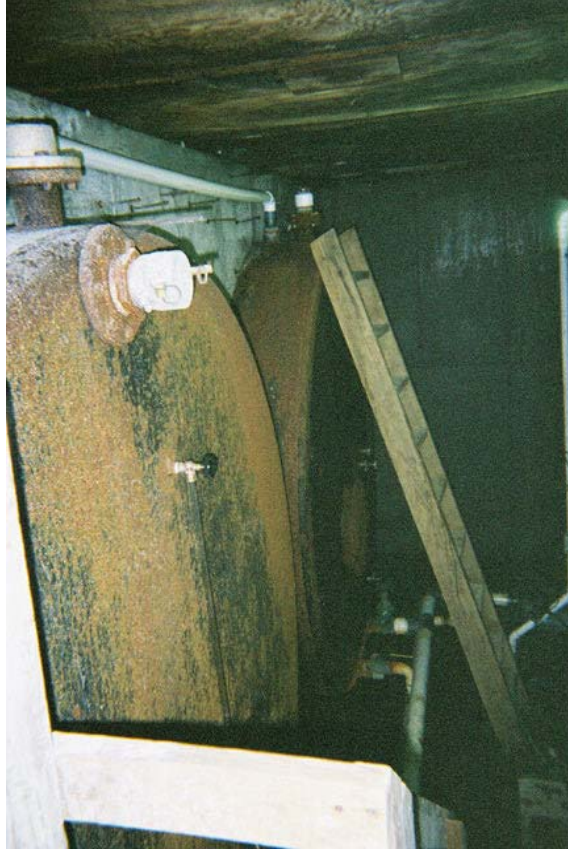
Figure 4-2. Preexisting Storage Tanks in Underground Concrete Structure
