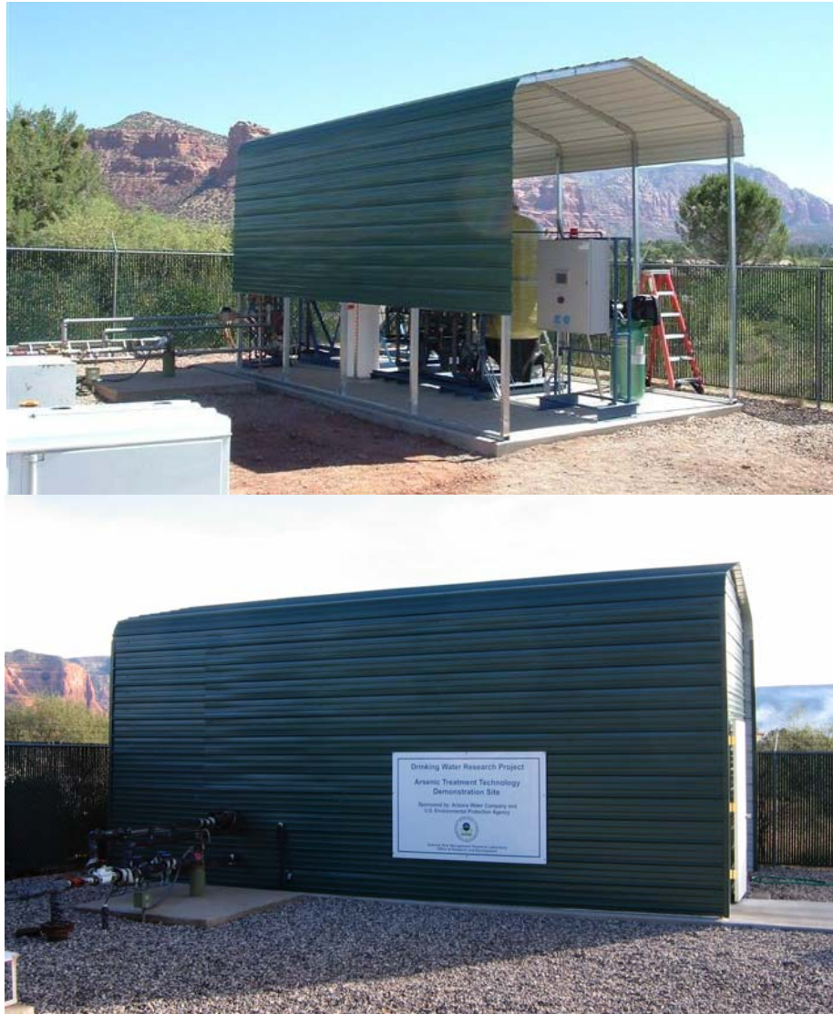
Figure 4-7. Sun Shed (Top) and Completed Enclosure (Bottom)
