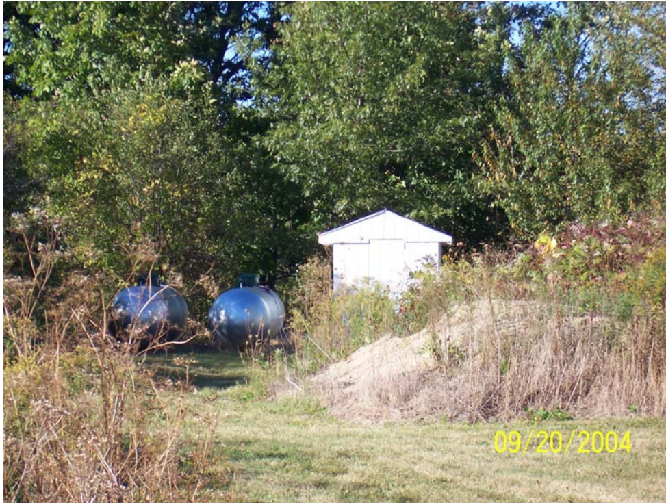
Figure 4-1. Preexisting Well No. 1 Pump House
