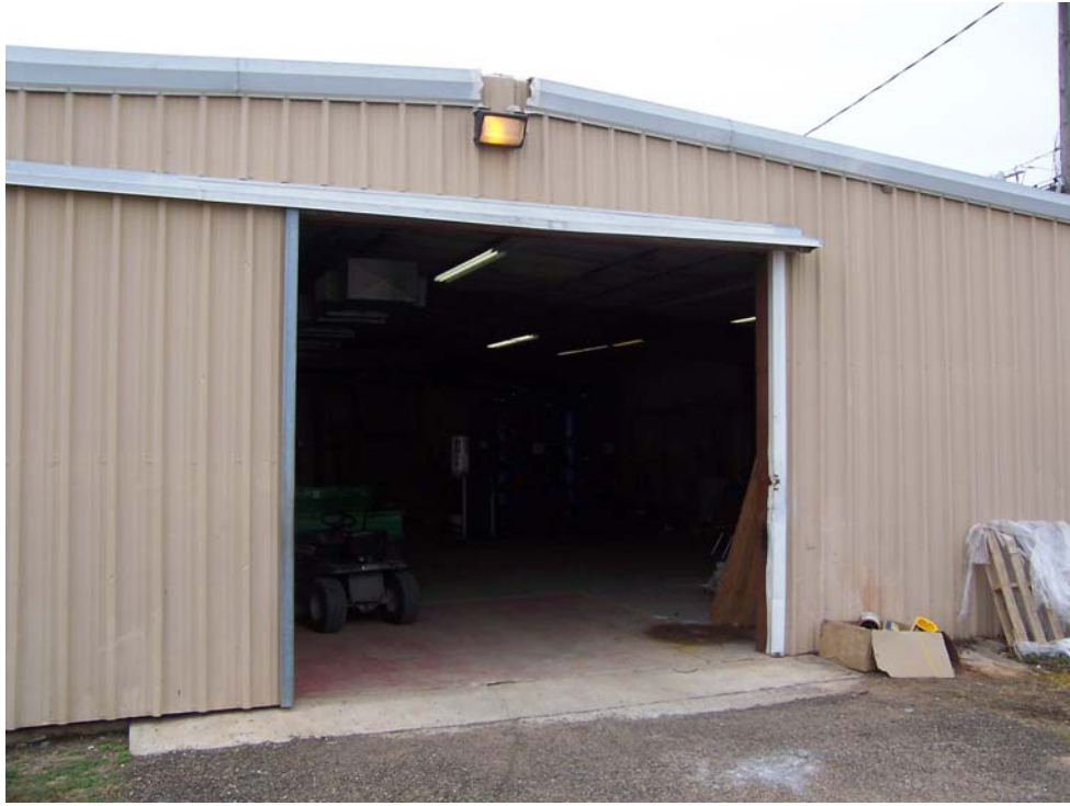
Figure 4-10. Maintenance Shop Building
