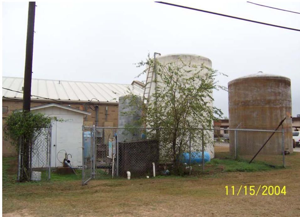
Figure 4-1. Existing Water Treatment Facility
