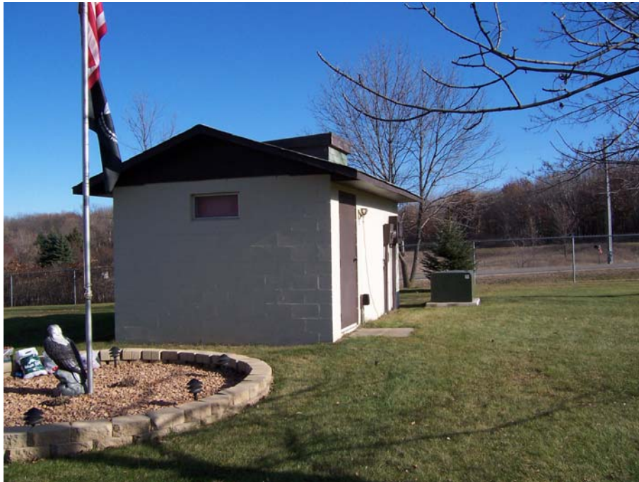
Figure 4-1. Pre-Existing Pump House at BSLMHP, MN Site
