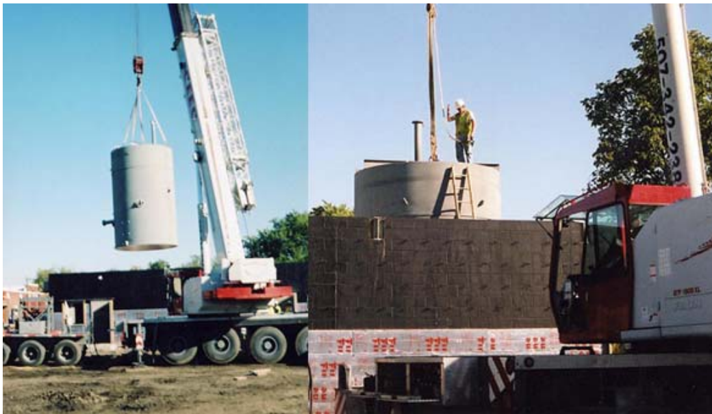
Figure 4-11. Off-Loading and Placement of AERALATER® Unit at Stewart, MN
