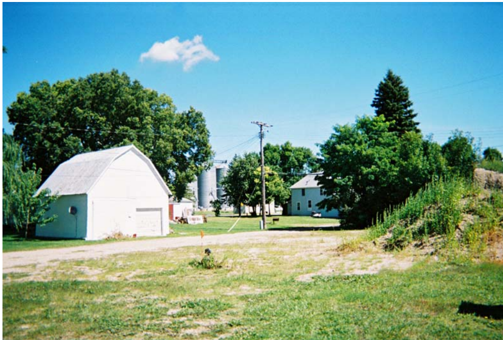
Figure 4-1. Wellhead 3 at Stewart, MN (near orange flag in center of photo)
