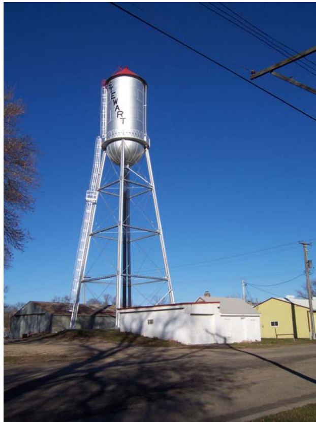
Figure 4-5. A 65,000-Gal Water Tower at Stewart, MN
