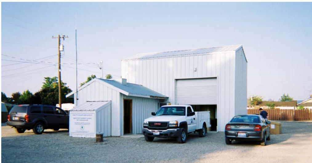
Figure 4-10. New Addition to Old Well House
