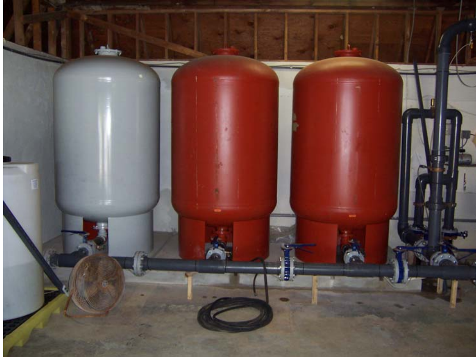
Figure 4-8. Hydropneumatic Tanks
