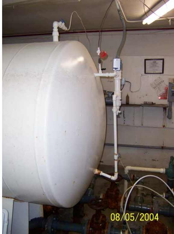
Figure 4-3. Pre-Existing Storage Tank
