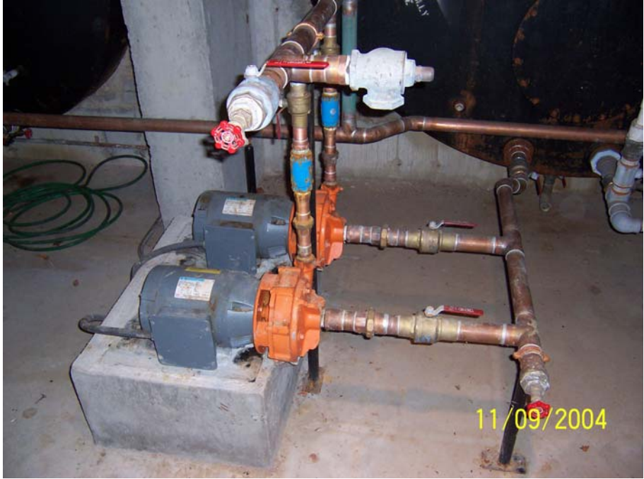
Figure 4-4. Booster Pumps
