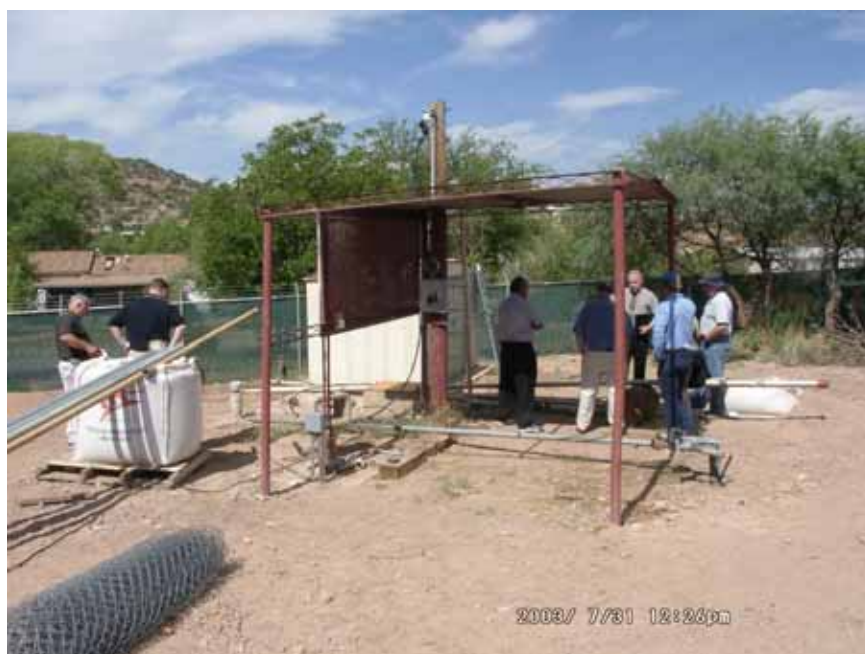
Figure 4-1. Pre-Demonstration Site Conditions
