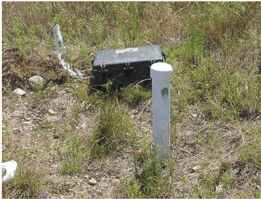
Passive Vent Gas Sampling
