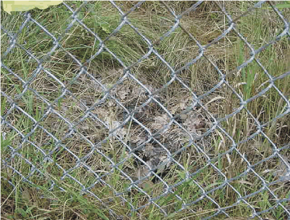
Storm Drain on Landfill Property
