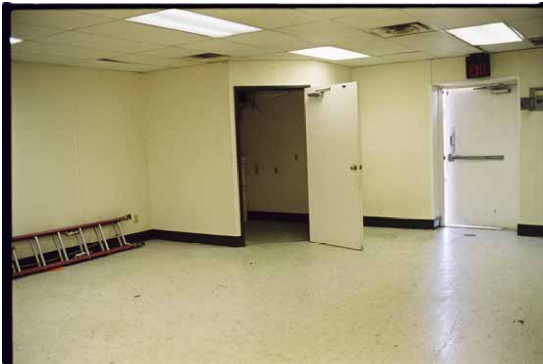
Figure 2-6. Back Room at Former Dry Cleaning Facility
