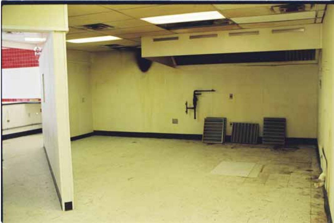
Figure 2-5. Fry Room at Former Dry Cleaning Facility
