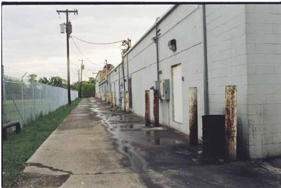
Figure 2-2. Back View of Former Dry Cleaning Facility
