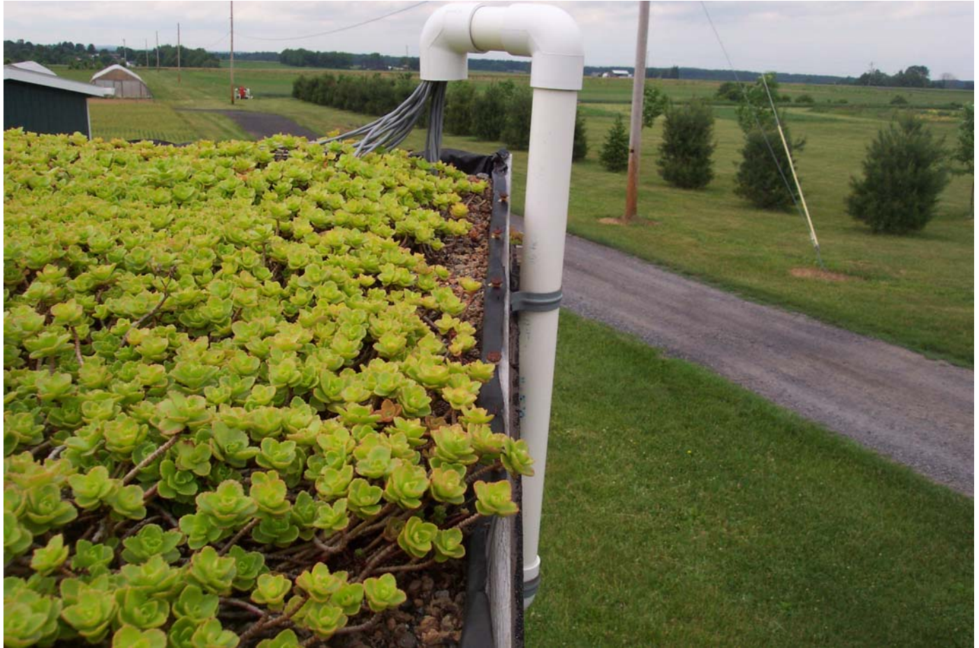
Figure A-4. Same green roof with monitoring equipment, June 2005
