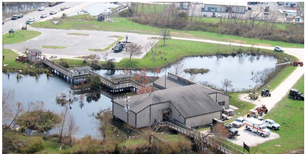
Cameron Prairie as Cameron Parish 911 Operation Center
