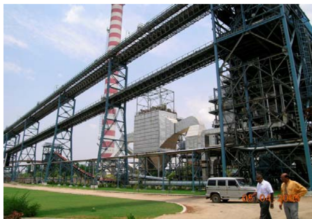
Godavri Sugar's 24 MW bagasse cogeneration plant in Karnataka, India, Photo: Sandeep Tandon
