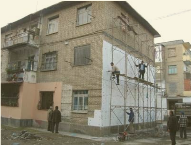
The façade of a building undergoing an energy efficiency intervention
