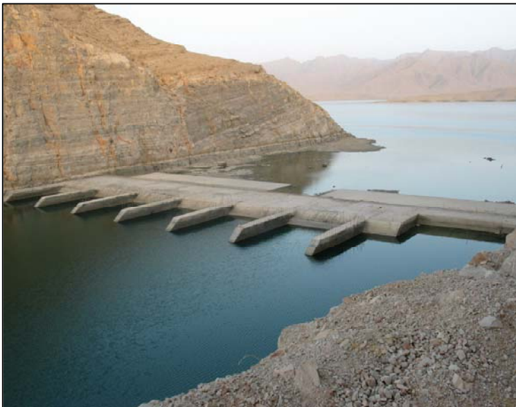
USAID is supporting the repair and expansion of the Kajakai Hydropower Plant to increase power supply to Kandahar and Lashkar Gah.
