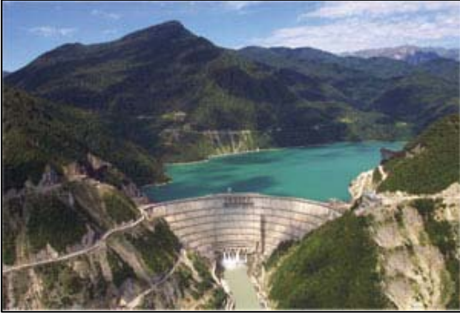
Enguri Hydropower Plant
