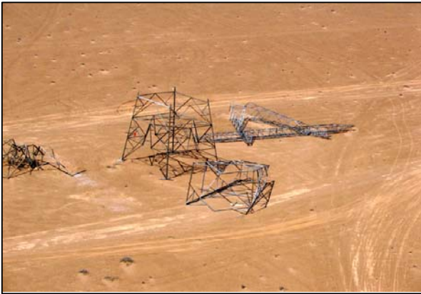
A downed transmission tower near the Thar Thar Canal
