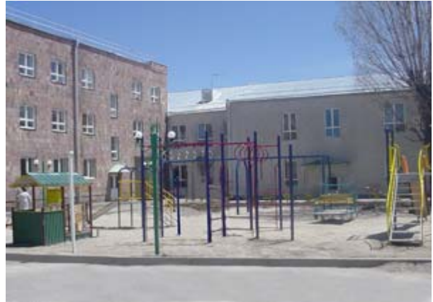
Heating system of this orphanage in Gavar town has been rehabilitated with USAID funding
