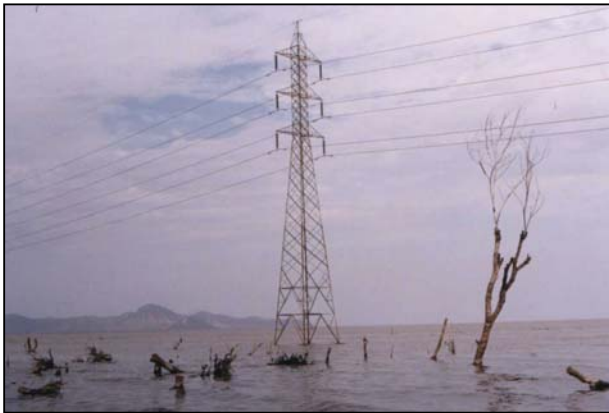
Electrical tower on the edge of Lake Managua
