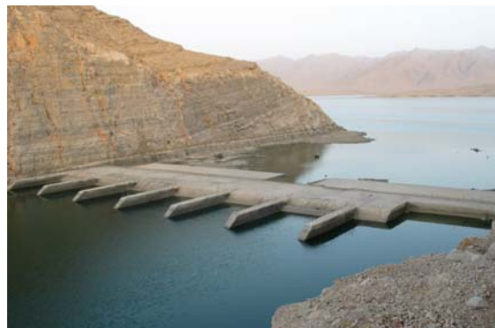
As part of the Afghanistan infrastructure program, the Agency will repair two Units at the Kajakai Hydropower Plant shown above, bringing electricity to 36,000+ people
