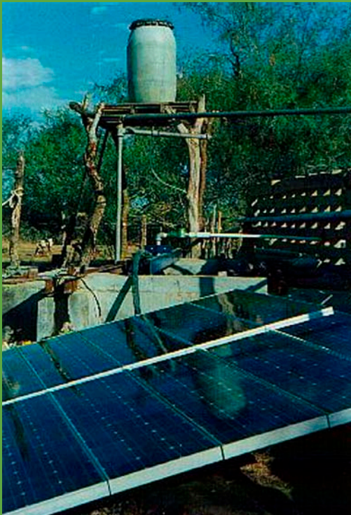
Solar powered water pumping system supports irrigation needs of farmers in rural Mexico.
