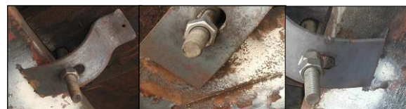
Figure 7a (left). HCP-25 Spring Clip with Single Nut. Figure 7b (center). Rotated Spring Clip and Gouge in Girder Flange. Figure 7c (right). HCP-25 Spring Clip with Double Nuts.
