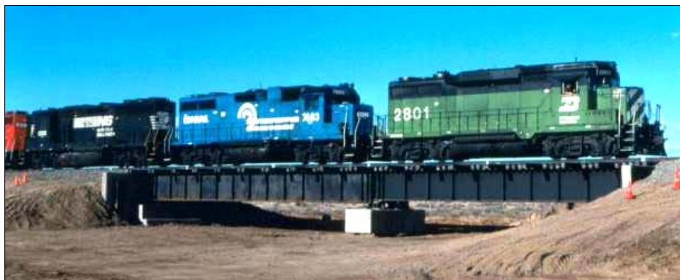
Figure 1. Open Deck Steel Bridge at FAST.
