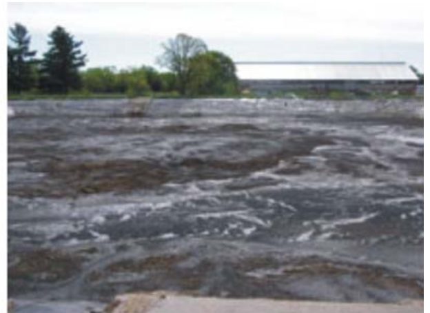
Figure 1. Lagoon showing sludge island before treatment and after collapse into the bottom of the lagoon.
