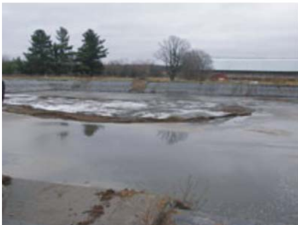
Figure 1. Lagoon showing sludge island before treatment and after collapse into the bottom of the lagoon.
