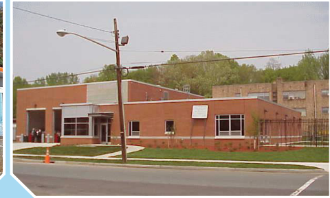
Site reused as a firehouse
