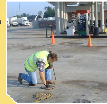
Inspecting a spill bucket
