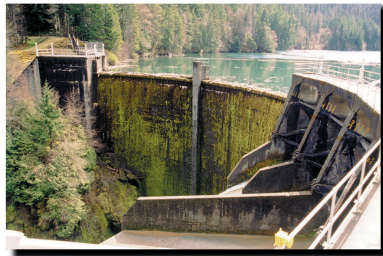
Safety of dam modifications consists of correcting identified structural deficiencies. These deficiencies could lead to a failure, resulting in uncontrolled releases of stored water that would place downstream populations and resources at risk (photo by BOR).
