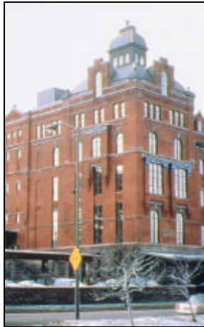
Stegmaier Building, Wilkes-Barre, PA
