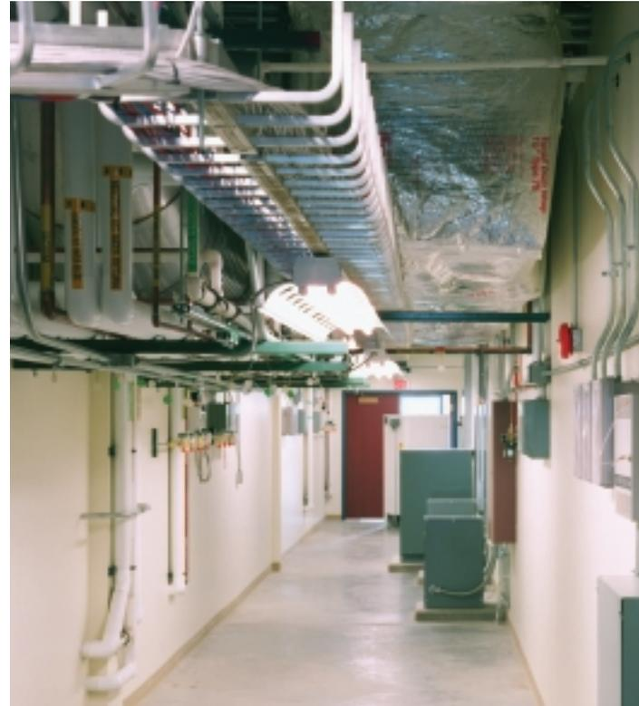
*Separated utility corridor provides minimal disruption for maintenance of mechanical equipment, electrical, and plumbing for laboratories.*
