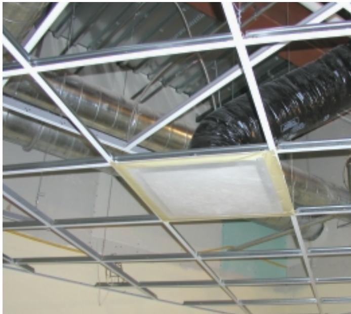
*During construction, the HVAC system and duct work were sealed on a daily basis to prevent infiltration of any dust, chemicals, or odors due to construction.*
