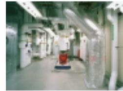
White pipes on right carry rain water drained from the roof.
