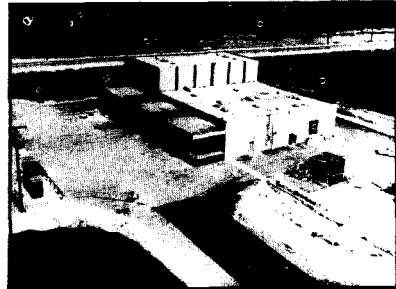
Figure 3.1.3 Fuel Preparation Building
