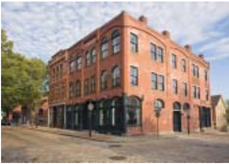
Newly renovated Corson Maritime Learning Center
