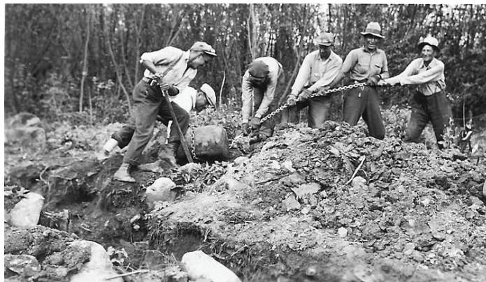
CCC-ID Grand Portage Stockade Excavation 1936. Taken by MHS archeologist Ralph Brown
