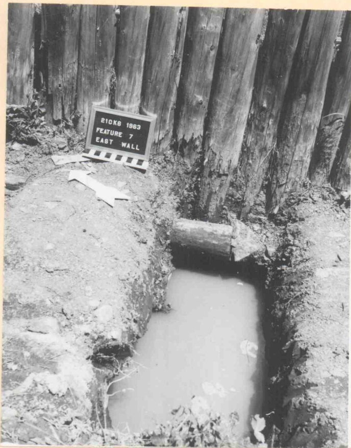
Water filled test pit
