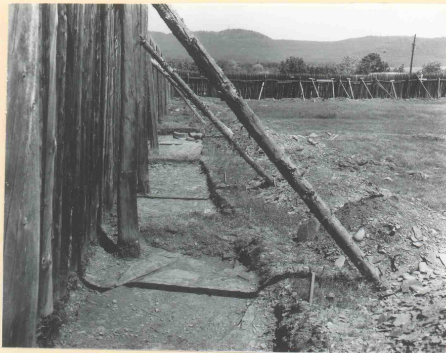
Excavation along interior of Northern palisade
