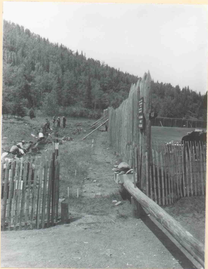
Excavations along exterior of Western palisade
