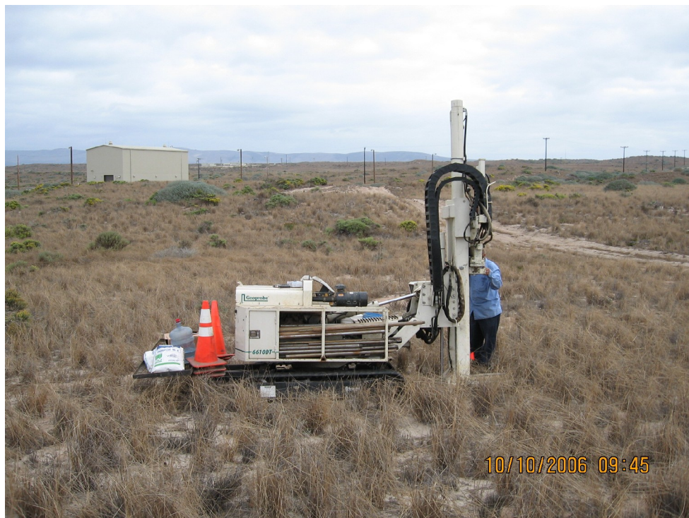
Photograph 2 – Drilling at location C1
