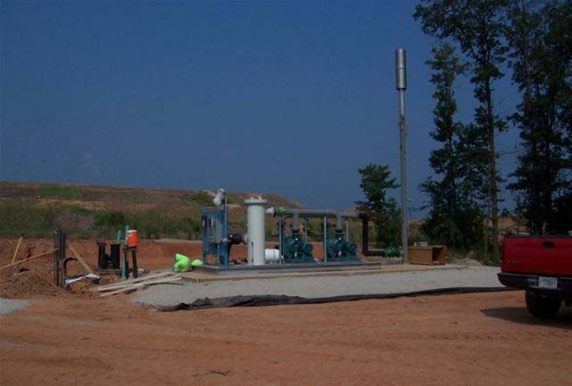
Construction of gas collection and combustion system at LaGrange landfill
