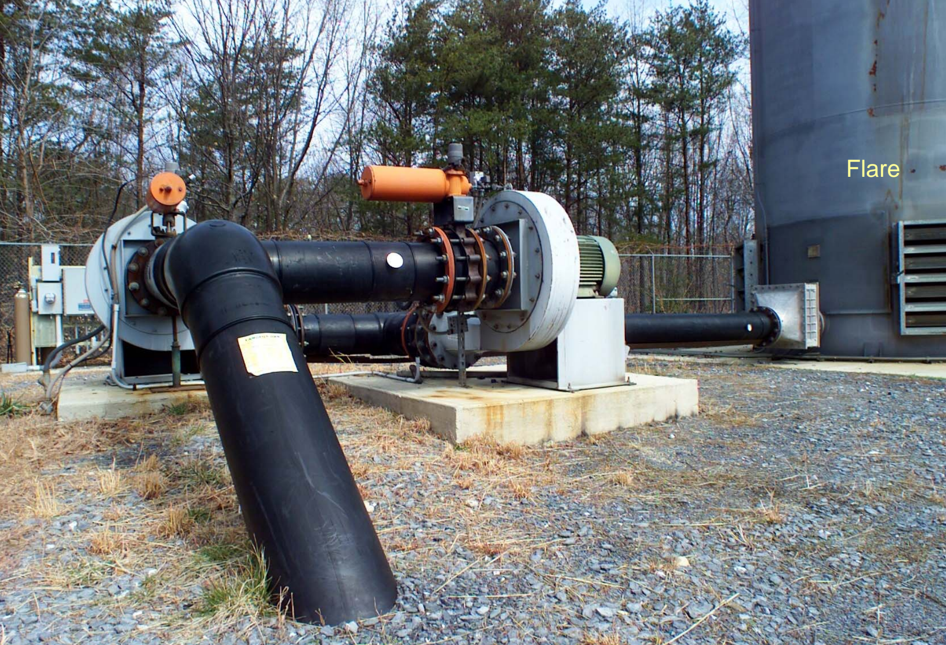
Pipes and flare installed for gas collection and combustion at LaGrange landfill
