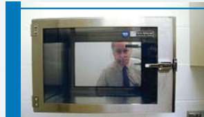
Sample Pass-Through Portal Sample containment is enhanced by the ability to pass samples from the Sample Reception Laboratory to the Analytical Laboratory through the Sample Pass-Through Portal.
