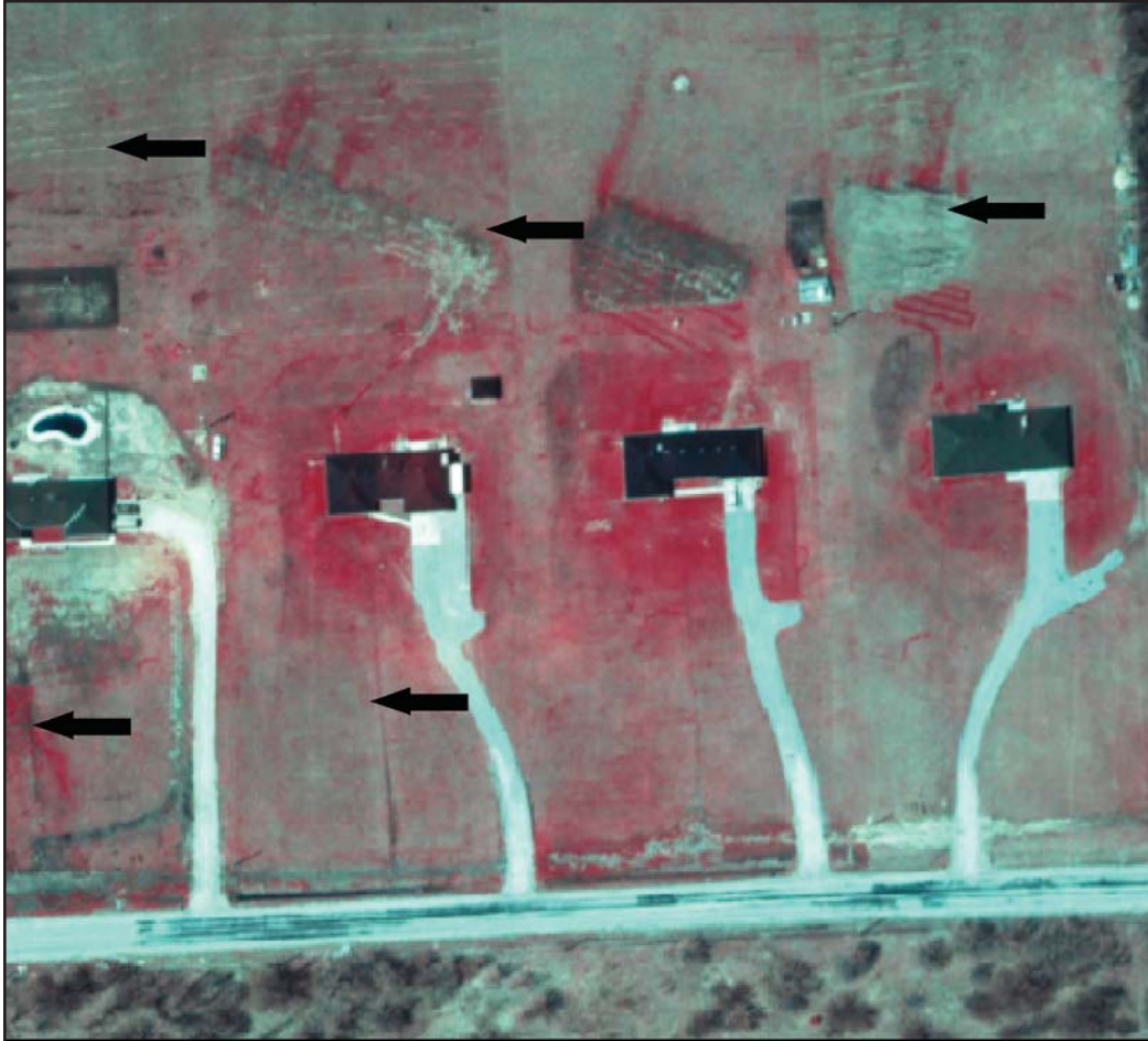
Figure 2. Secondary signatures. This false color infrared photo shows the common practice of covering a failing absorption field and rerouting wash water through small ditches.
