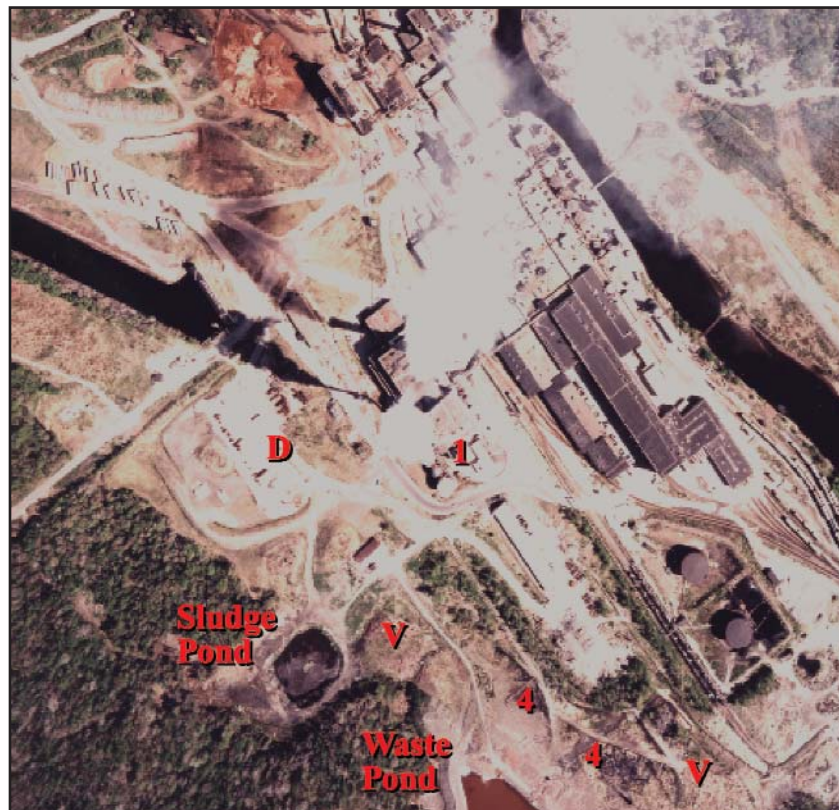
Figure 1. Photo and site analysis for an SPCC report, showing spill conditions.
